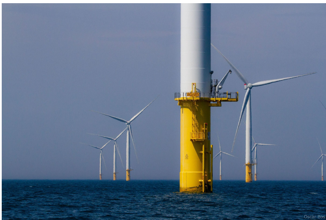
Figure 2. Turbine W5 in Gemini offshore windfarm.
