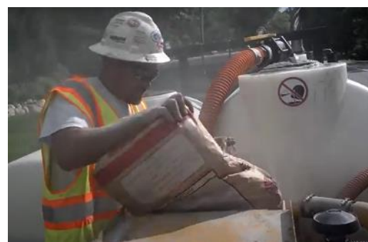
Figure 16: Conventional mud mixing: add bags manually to a mix hopper
