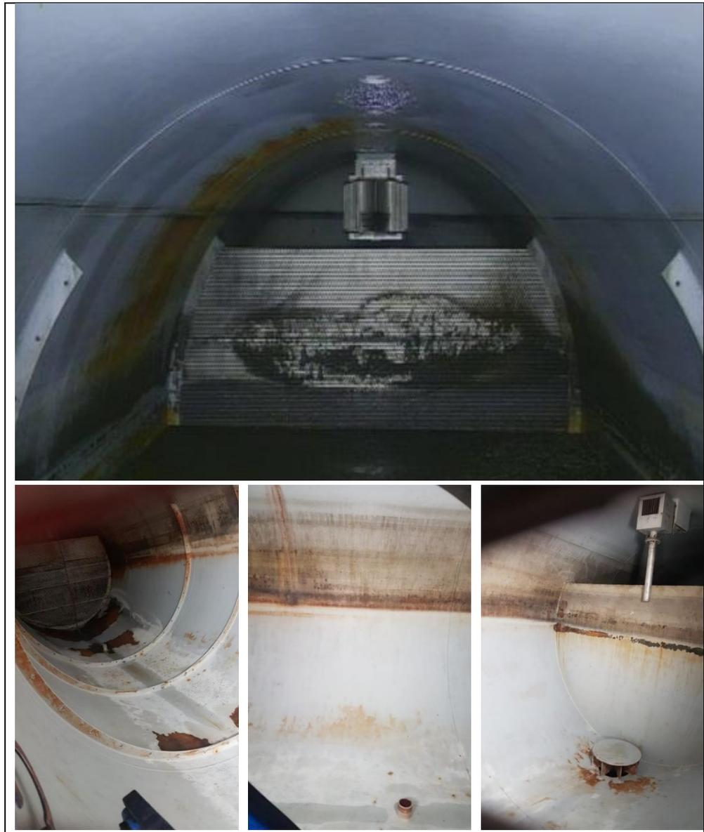
Figure 14 - Damage found by ECW during one of prescribed 4-yearly inspections of the separator.
