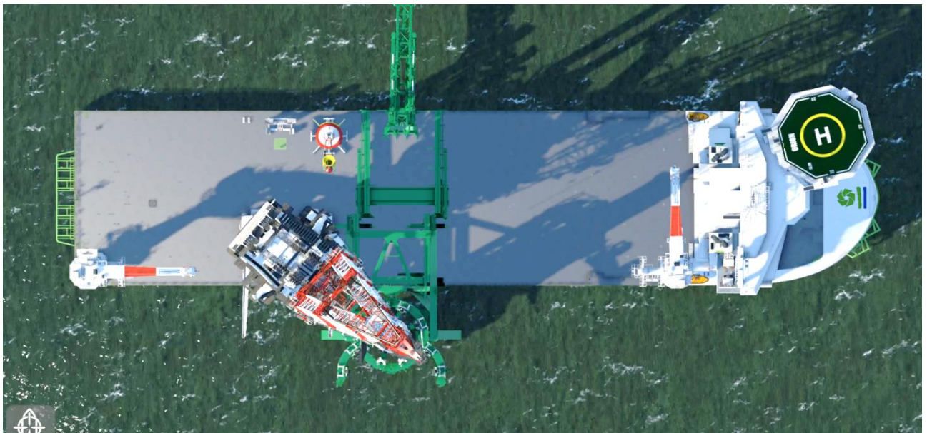
Figure 6-4: Step 3: motion compensated piling phase
