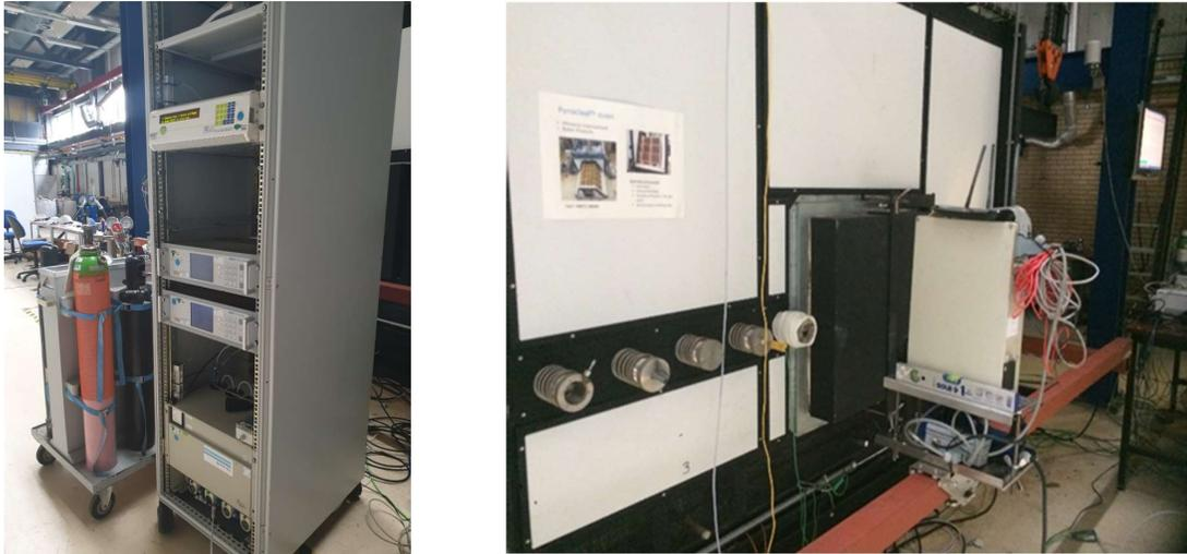
**Figure 3.2: Analyzers for detecting  $\text{NO}_x$  and  $\text{O}_2$  in the flue gas (left). In-situ IR laser for detecting  $\text{O}_2$ , CO, water and the temperature in the furnace (right).**
