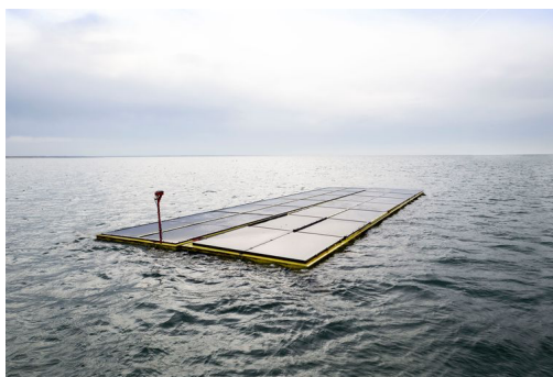
Figure 1 – Photograph of the offshore floating PV system developed by Oceans of Energy in the NS1 subsidy project “Zon op Zee” (TEHE117022) (© Oceans of Energy).
