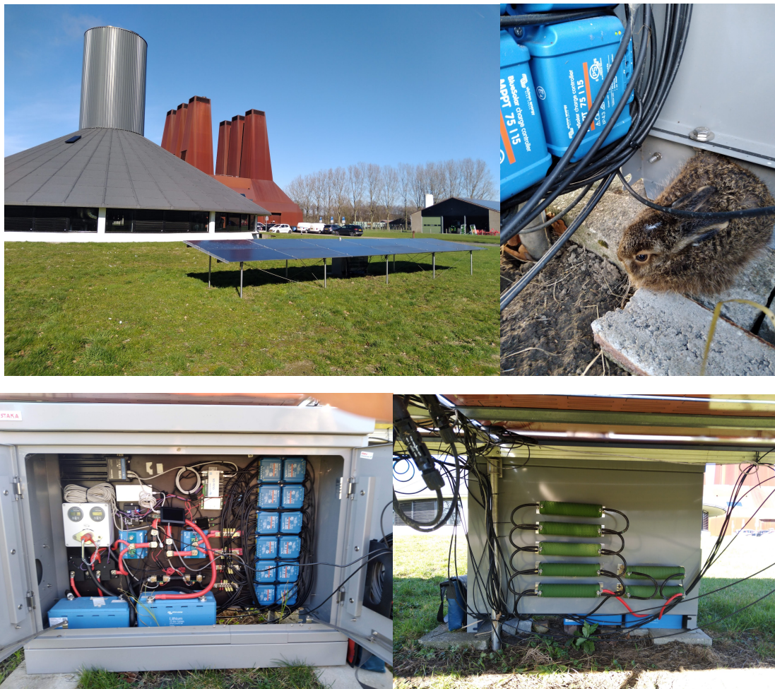
Figure 2 – Land based PV system, with cabinet for power optimizers, batteries, and energy management system, with dump loads on the back. Local wildlife used it as refuge.
