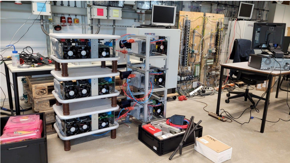
Figure 21 Prototype testing at TU/e – complete AC/DC and DC/DC stage of the converter
