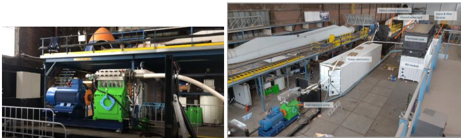
FIGURE 3 DOT WORKSHOP TEST SETUP (PHASE 1 & 2)
