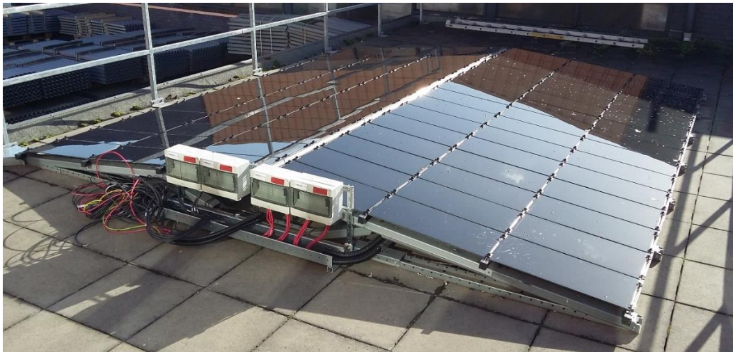
Figure 7: Test roof based on thin film roof tiles.
