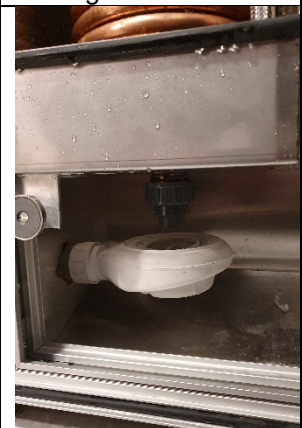
Montage airbreak to drain
