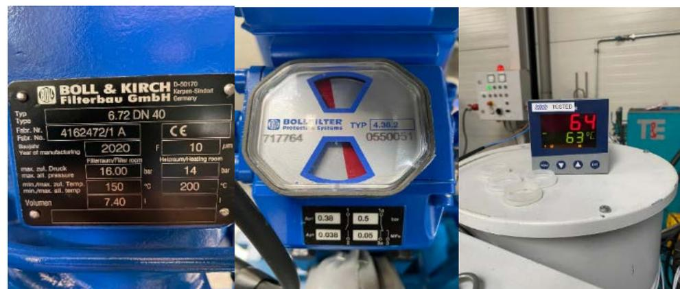
Figure 50 Specifications left photo) of a dedicated filter for shipping fuel and indications for filter clogging (right two photo's)
