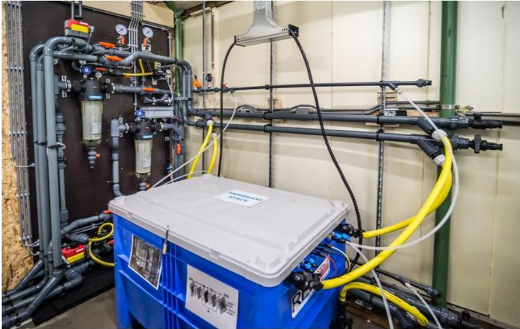
Fig. 1: Pump and filter system (at the wall panel) and two stack boxes. Per blue box two membrane stacks are present, together being able to generate 200 Watt power. Above the box three cables (grounding, phase and switch wire, combined in black wrapping for safety purposes) go into the cable tray, from both stacks. Piping work in the background supplies water to the two stacks, with two big pipes on top directing it back towards the reservoirs. Piping work will be extended to the right side in stage 2. The large piping work construction mounted on the concrete plex houses two big filters for fresh and salty water streams (to remove larger particles such as glue, saw dust, etc.), 3-way valves (red-yellow boxes), pressure meters (white clocks), and pumps (in-between the yellow tubing blue pumps are visible for fresh and salt water).
