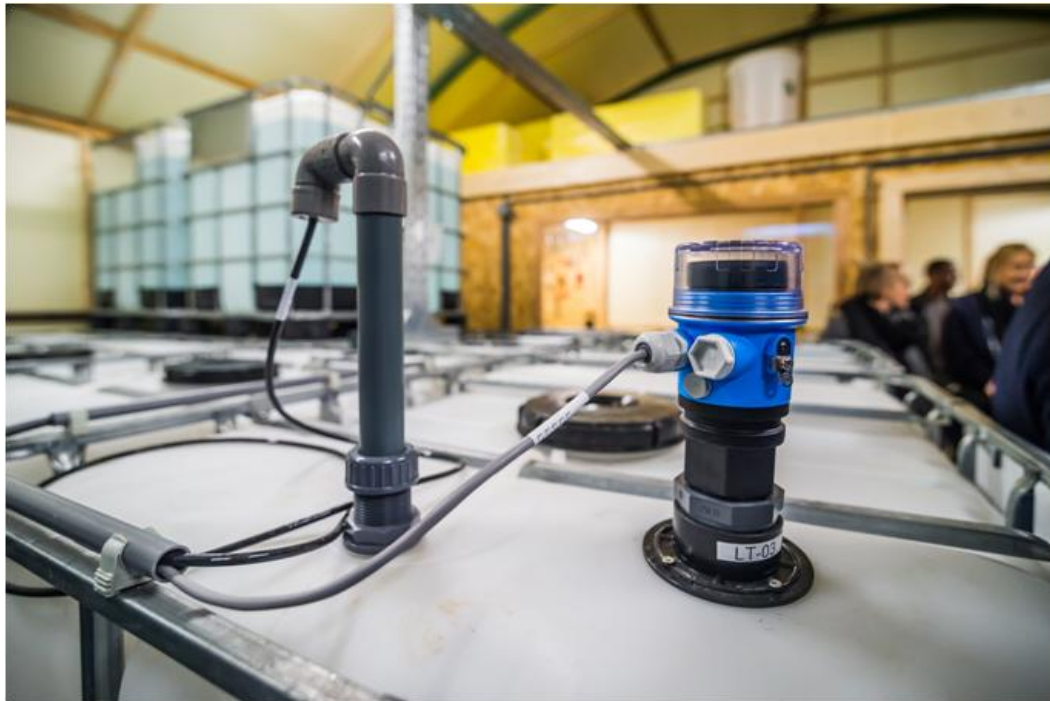
Fig 3: Close-up of the sensors. In the background the cable tray coming from IBCs is visible, installed for guiding the cables from sensors towards the electrical cabinet. Furthermore the control room is visible, below the big yellow blocks of insulation material. Installed in a separate room to have a 100% dry room for electrics and electronics, but also be able to heat up the place a bit for comfortable working on the BMS programming.
