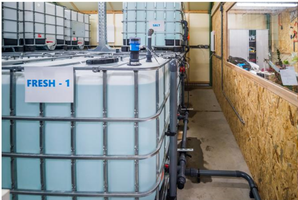
Fig. 1: Pump and filter system (at the wall panel) and two stack boxes. Per blue box two membrane stacks are present, together being able to generate 200 Watt power. Above the box three cables (grounding, phase and switch wire, combined in black wrapping for safety purposes) go into the cable tray, from both stacks. Piping work in the background supplies water to the two stacks, with two big pipes on top directing it back towards the reservoirs. Piping work will be extended to the right side in stage 2. The large piping work construction mounted on the concrete plex houses two big filters for fresh and salty water streams (to remove larger particles such as glue, saw dust, etc.), 3-way valves (red-yellow boxes), pressure meters (white clocks), and pumps (in-between the yellow tubing blue pumps are visible for fresh and salt water).
