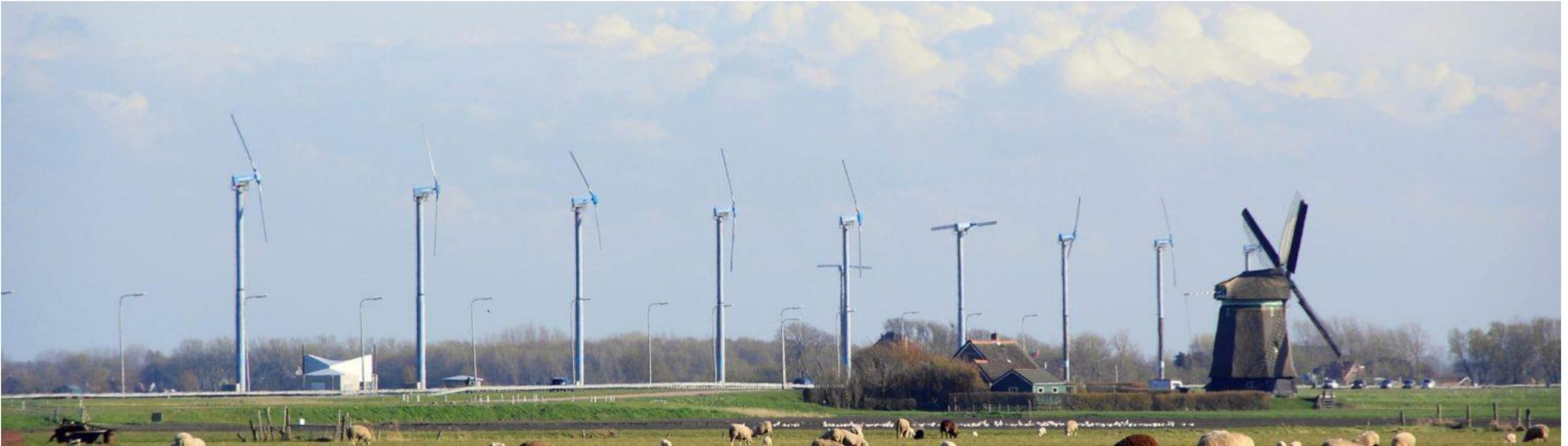
Originally 15 Lagerwey 15/75 turbines (75 kW)
