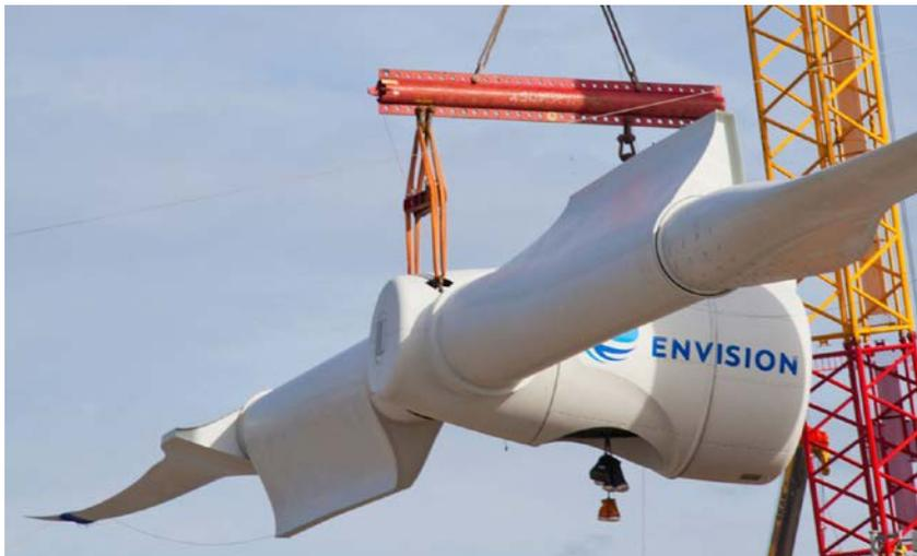
**Figure 16: rotor blade with pitch bearing at ca. 23m rotor radius (blade length 63m) [20]**
