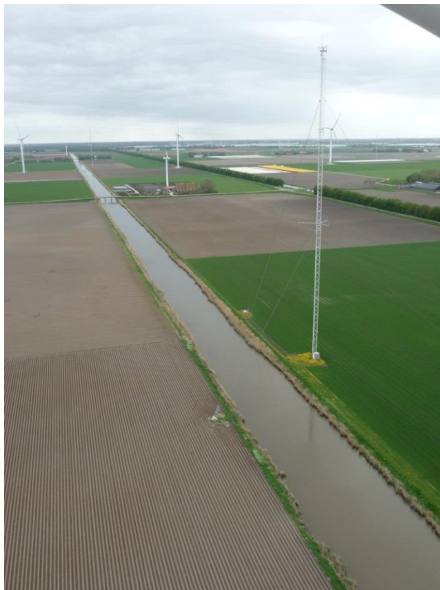
Figure 6-4: Photograph of MM3 at the EWTW test site, taken from N6
