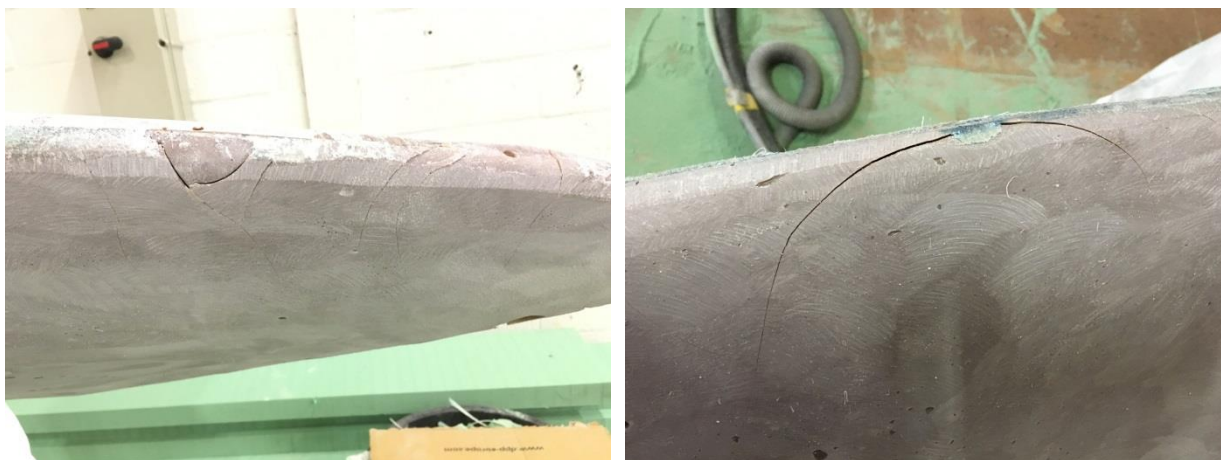
Figure 5-23: Glue cracking as seen after extreme load test
