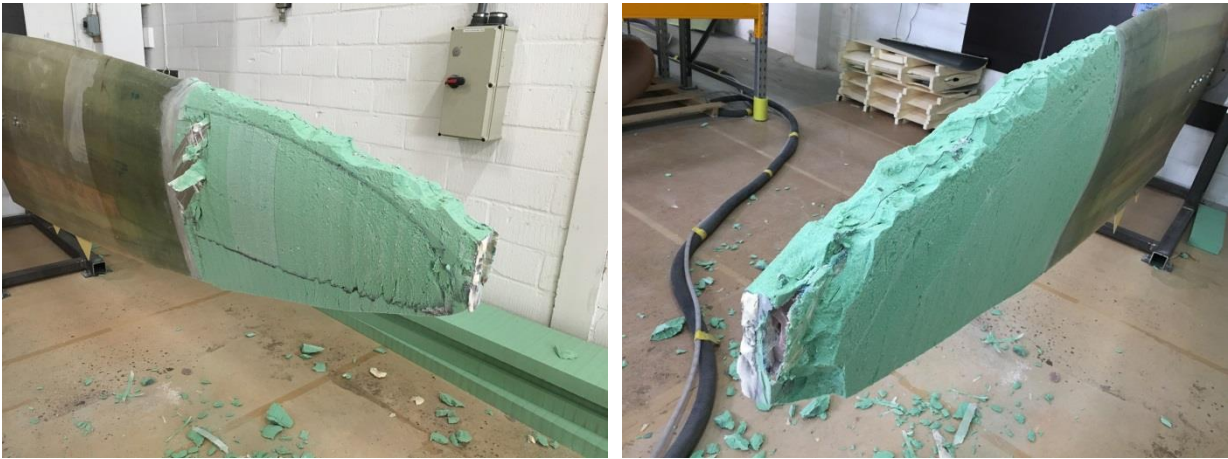
Figure 5-21: Removal of tip by cutting away tip, leading edge and trailing edge – grinding the connection and removing the glass cover
