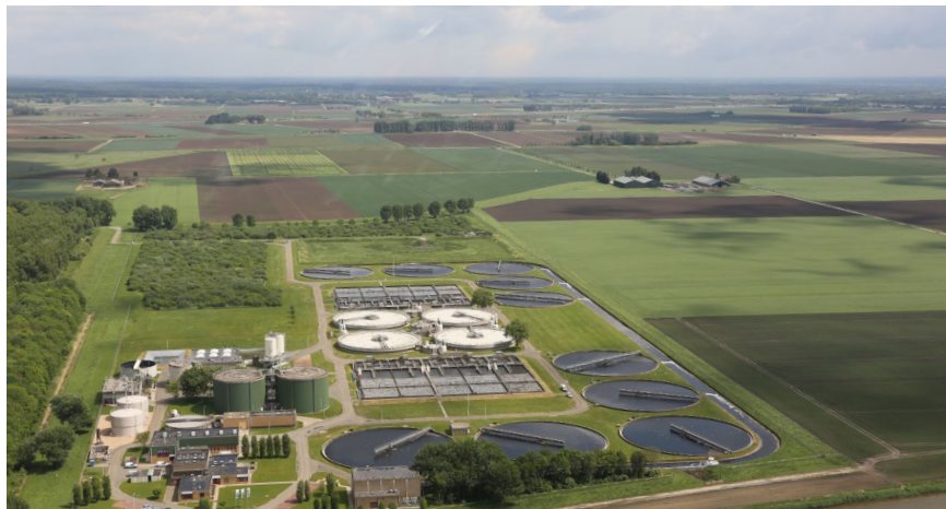
FIGURE 2 MUNICIPAL WASTEWATER TREATMENT PLANT BATH. THE PLANT TREATS WASTEWATER FROM 500.000 PEOPLE EQUIVALENTS AND HAS THE POTENTIAL TO SUPPLY BIOMASS TO PRODUCE 2000-2500 TON PHA/YEAR.
