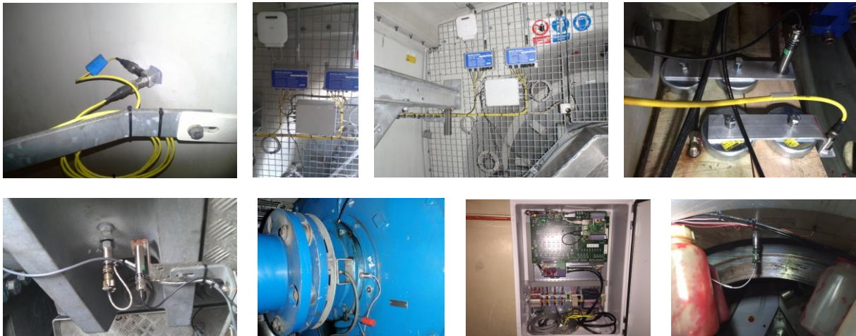
DAISY4OFFSHORE components installed
