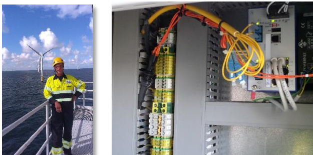
DAISY4OFFSHORE installed at Amalia
