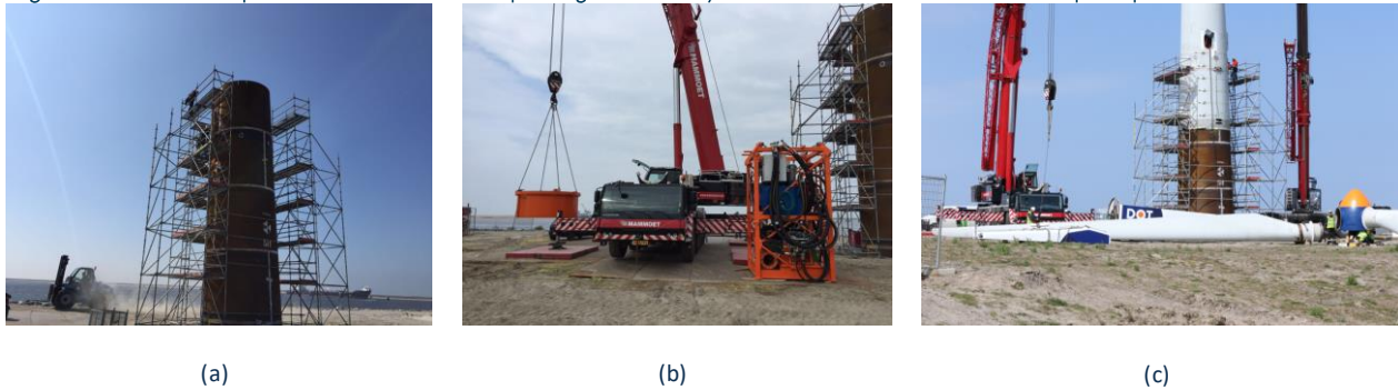
FIGURE 3 | SLIP JOINT INSTALLATION PROCESS
