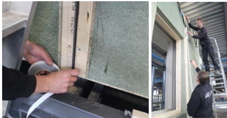
5. Airtight sealing between the panels
