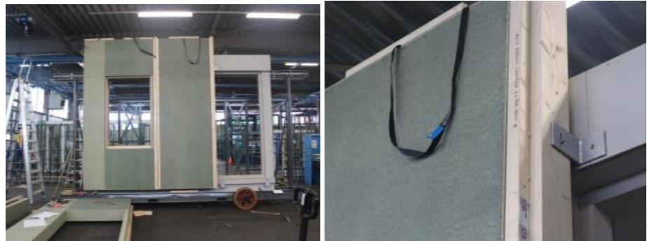
3. Central panel attached to the sub-structure, through timber sticks
