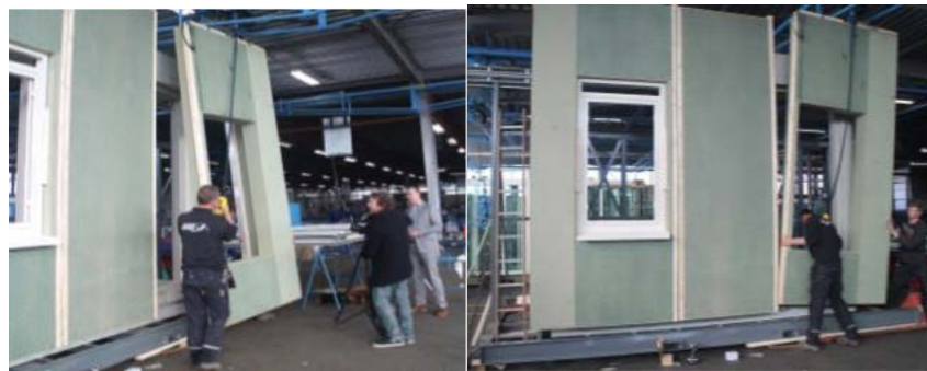
4. Left and right panel attached to the sub-structure, through timber sticks
